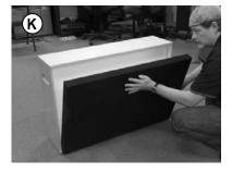
Before final assembly, the glue should dry completely. Temporarily install the acoustic panels to ensure the frame is square as it dries. Do not remove the protective plastic. It will prevent excess glue from sticking to the fabric.
